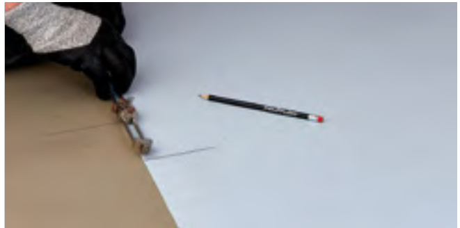
Figure 38 Scribing the wall profile
