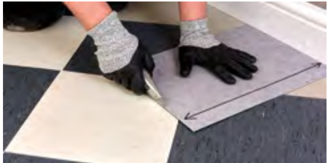
Figure 8 Cutting the perimeter tiles (diagonal cut)
