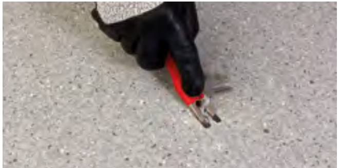
Figure 5b Final trim after the weld has cooled (Mozart Trimming Tool)
