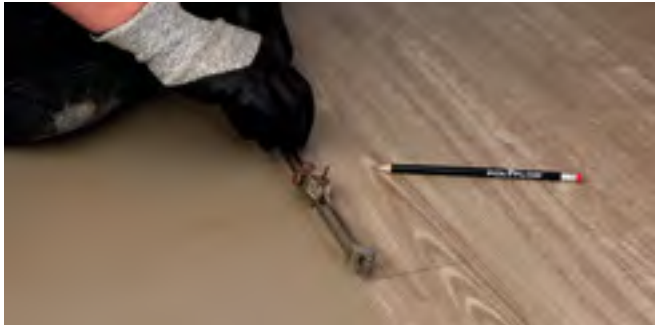
Figure 4 Scribing the wall profile
