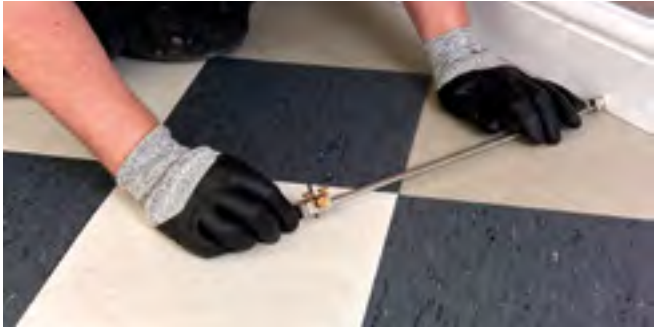
Figure 9 Cutting the tiles using a scriber (diagonal cut)
