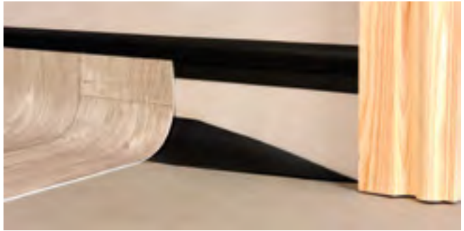
Figure 7 Taper towards a doorway
