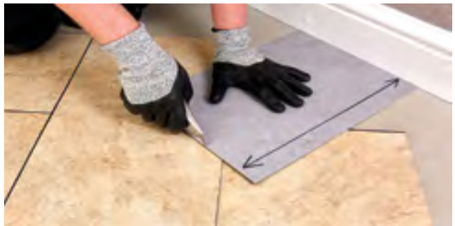
Figure 9 Cutting the perimeter tiles (diagonal cut)
