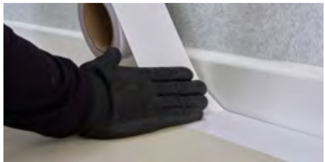
Figure 36 Use double sided QuickLay tape
