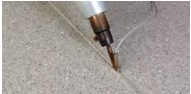
Figure 2 Applying the weld
