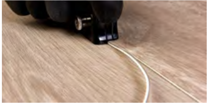
Figure 5 Cutting in the seams
