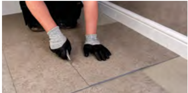
Figure 8 Measuring using an overlapping tile
