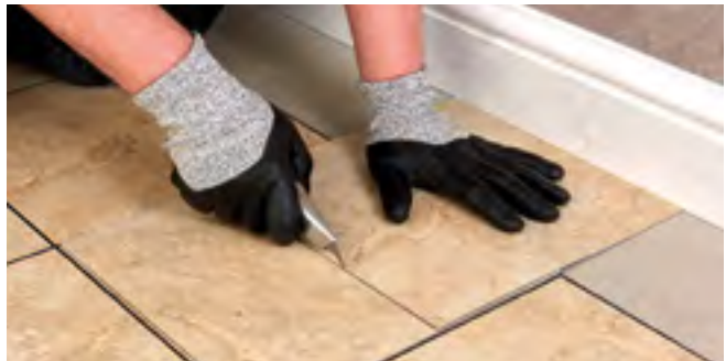
Figure 6 Measuring using an overlapping tile
