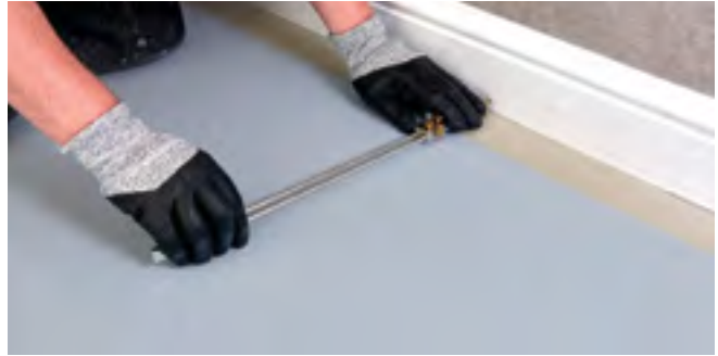
Figure 35 Scribing the wall profile
