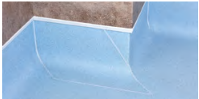
Figure 11 External corners 'wrap around method'
