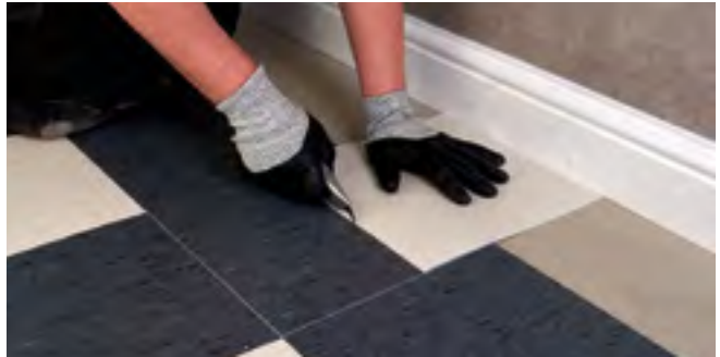
Figure 5 Measuring using an overlapping tile
