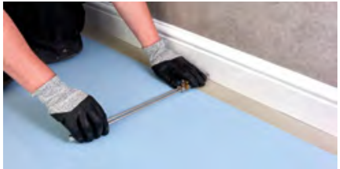
Figure 2 Scribing the wall profile
