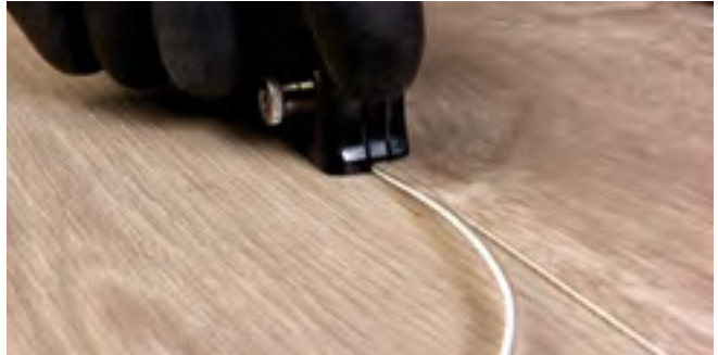
Figure 5 Cutting in the seams
