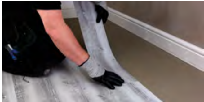
Figure 1 Setting planks out
