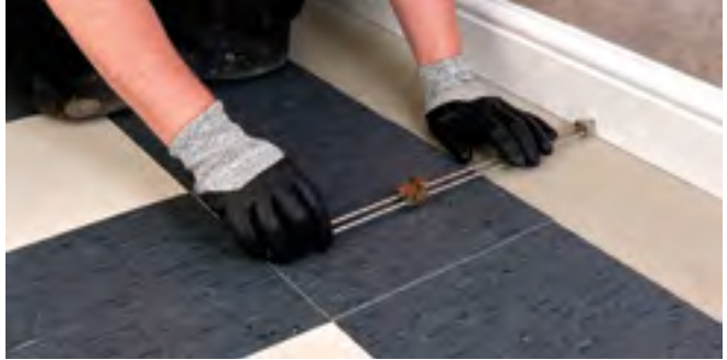
Figure 6 Measuring a tile using a scriber
