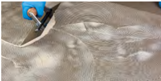
Figure 6 Spread the adhesive
