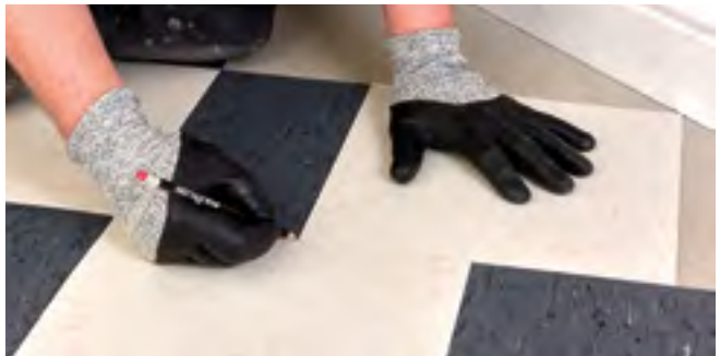
Figure 7 Marking the perimeter tiles (diagonal cut)
