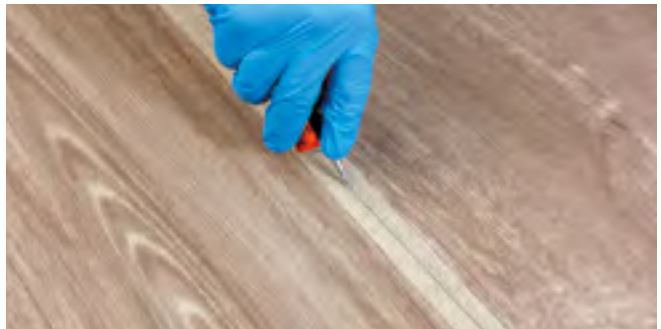
Figure 7 Cold welding
