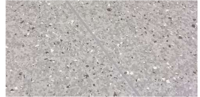
Figure 9.6 Final weld
