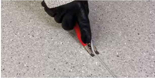
Figure 9.4b Trimming off the weld top layer (Mozart Trimming Tool)
