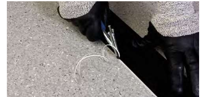
Figure 9.1 Grooving the seam
