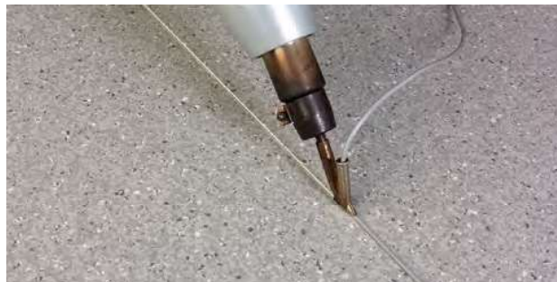
Figure 9.2 Applying the weld
